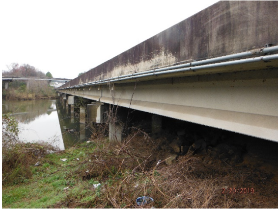
Photo 1. East View of Bridge
