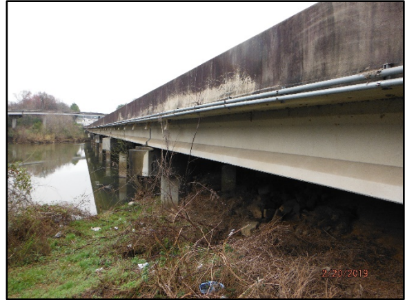
Photo 1 – I-26 Bridge over Saluda River in Richland/Lexington, SC.
